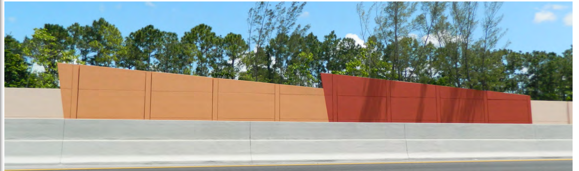
EXAMPLE OF NOISE WALL "C" SR 874 CORRIDOR
