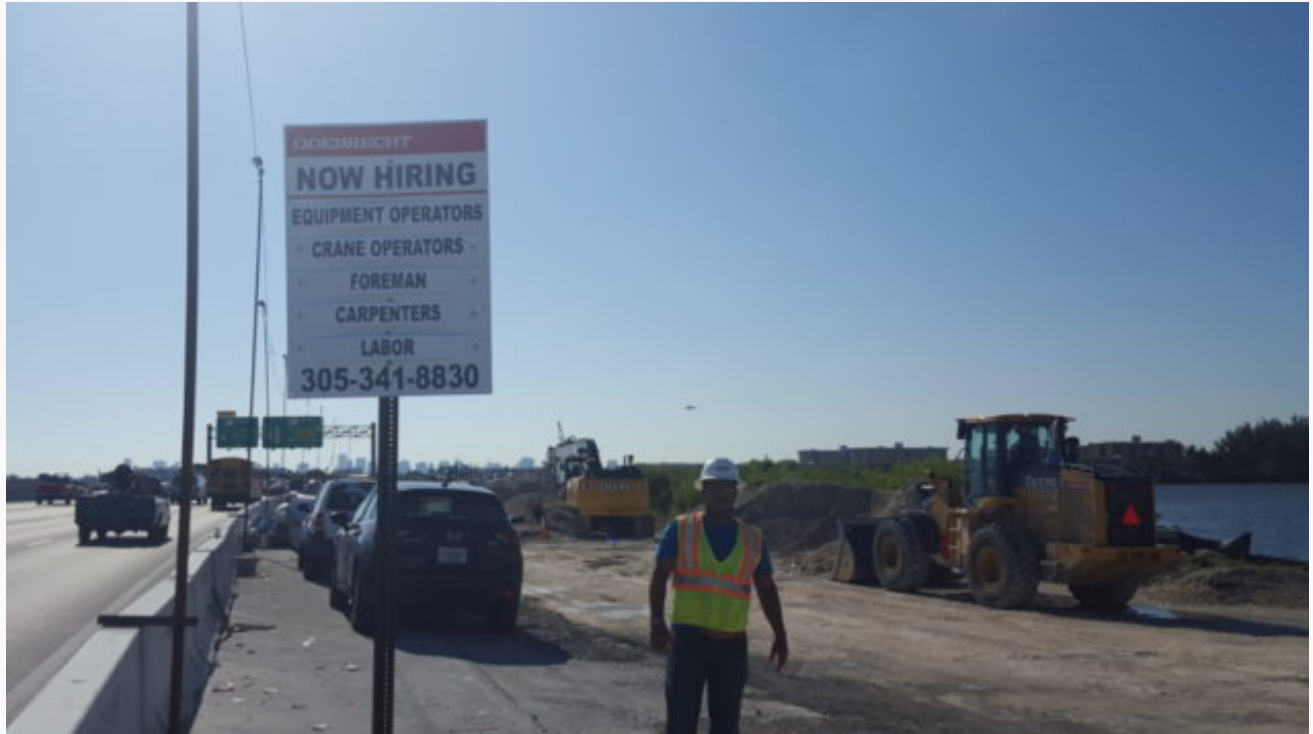
Odebrecht Construction is under contract for two MDX project along SR 836
